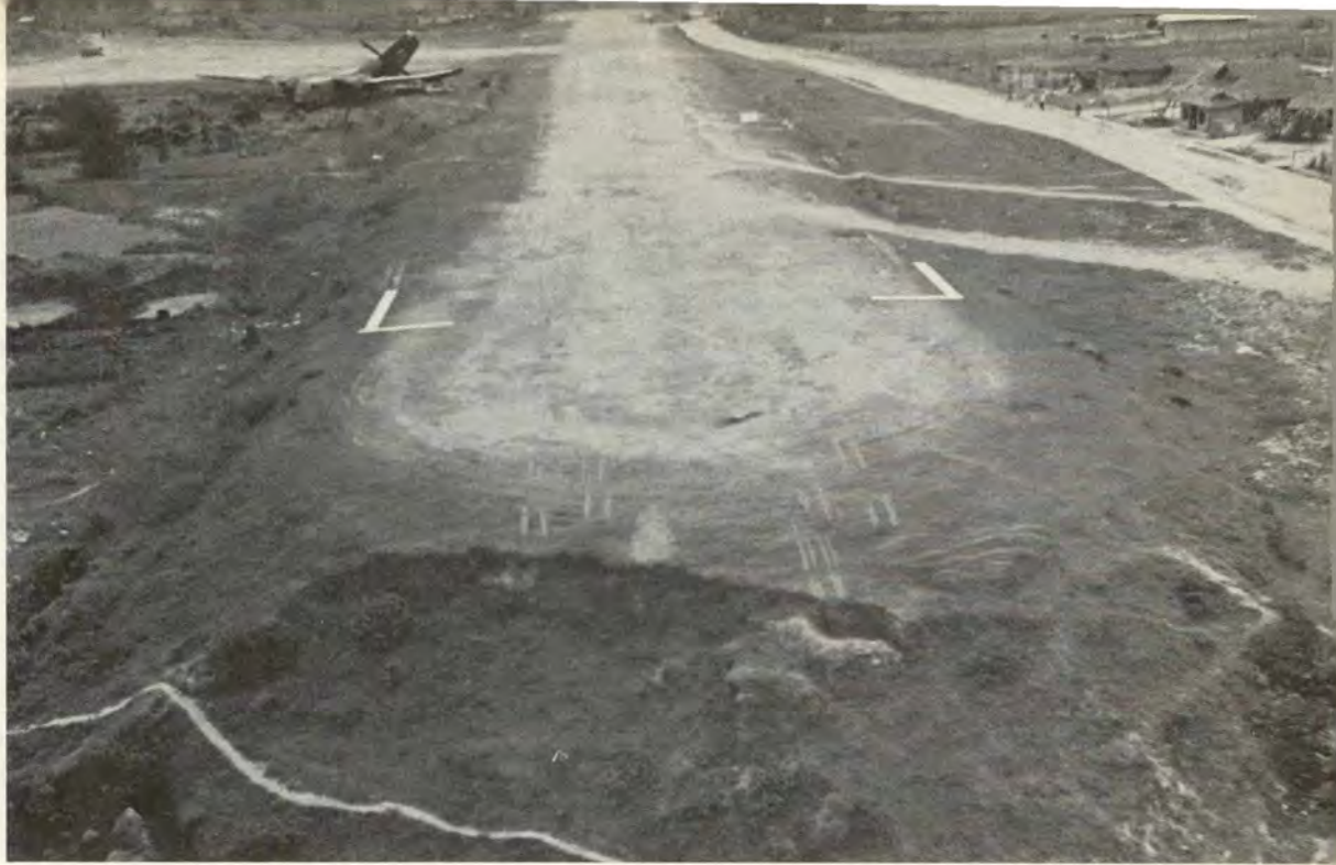
Tire marks indicate where wrecked C-7 (upper left) touched down on lip of slope. Runway is 1100 feet long, white rectangle on right side is 200 foot marker.
